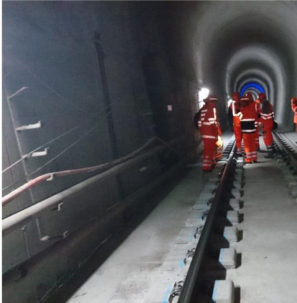
16 bridges, 24 culverts, 94 retaining structures and 9 tunnels are being refurbished on the 12-kilometre stretch between Brunnen and Flüelen. SBB is renewing the superstructure along the entire route – with some use of the slab track system in tunnels. In the tunnels, overhead contact lines are also being replaced by overhead conductor rails, arches and walls are being reinforced and replaced, new cable systems are being constructed and self-rescue facilities such as alcoves are being installed.
